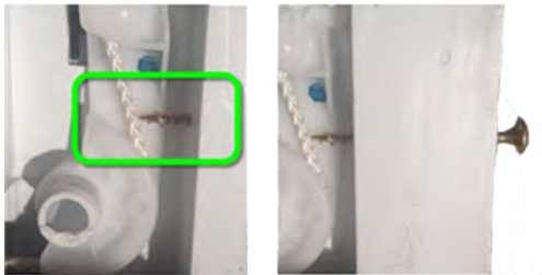
Fig. 26: Consequences of not using supplied toe panel screws
