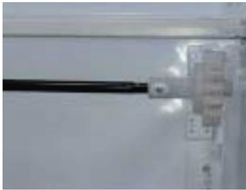
Step 4) Insert opposite gear ice into connector rail and screw them
