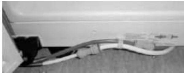
DRAIN PIPE ASSEMBLY
